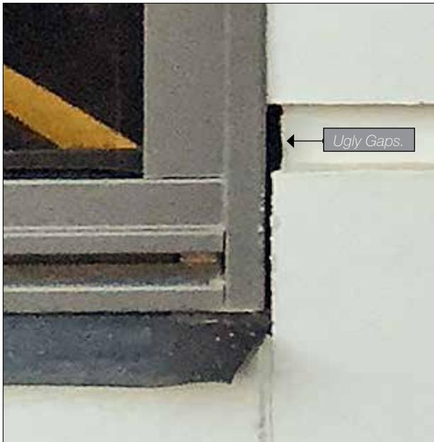
**Traditional Finish:** Cladding is tucked in behind the external leg of the window frame.
