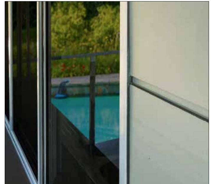
**CLAD-TRIM:** The **P14995** and **P14996** are factory fitted to a selected range of Dowell products and provide a neat finish and easy access for caulking/sealing the boards.
