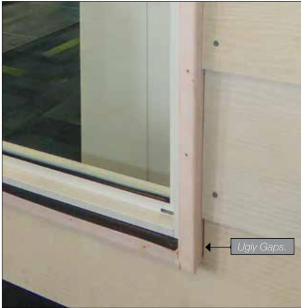
**Picture framed finish:** Timber used varies in size depending on cladding selected and the desired finish.
